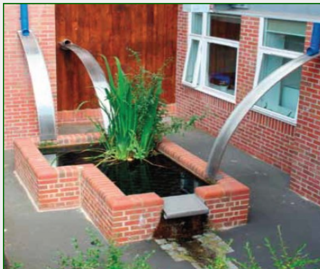
Fort Royal Primary School, Worcester – three rain slides deliver roof water into a raised pool which overflows into a set channel and rill before flowing to a wildlife pond in green space, all accessible by children. Photo: Bob Bray
