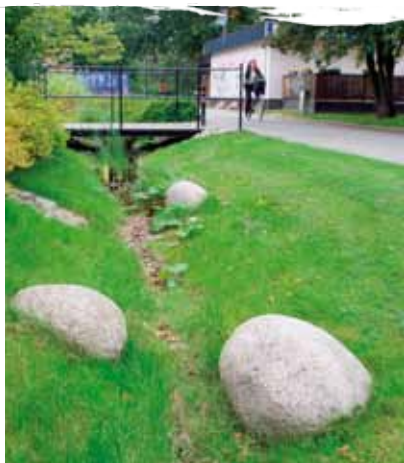
Augustenborg, Malmö, Sweden – an open swale next to a cycle route with large boulders common in many Swedish landscape designs showing a confident approach to risk. Photo: Bob Bray
