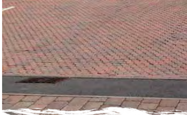
Fort Royal Primary School, Worcester – block paving is one of a number of permeable surface types facilitating water filtration into the ground below or collection chamber. Photo: Bob Bray
